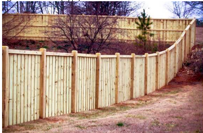
Figure 40.1-5.10(K)(2): Fence Finished Side to Outside
